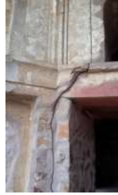
Figure 25: Vertical Crack
