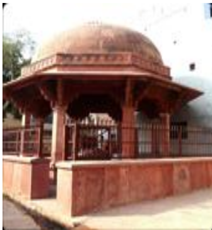
Image 5.2.12 External view of Barah Khamba
