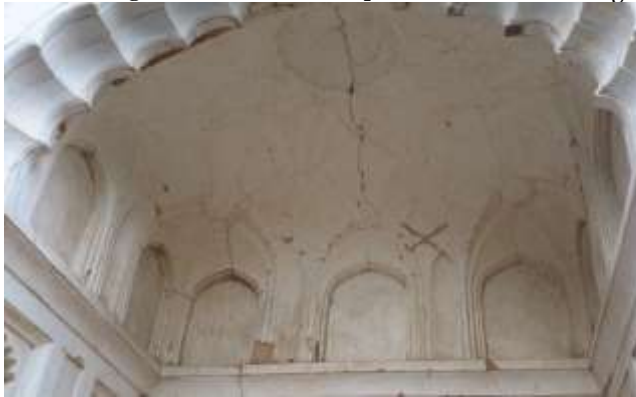
Figure 51: Structural Crack
