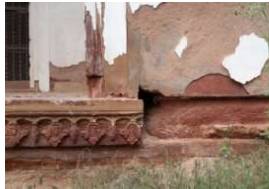
Figure 52: Openings at Base
