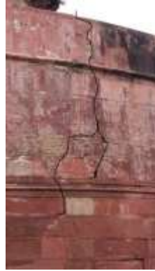
Figure 22: Vertical Crack
