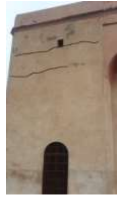
Figure 31: horizontal crack
