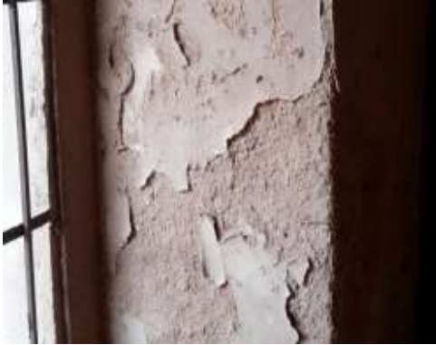
Figure 57: Plaster removal
