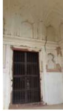
Figure 49: Vertical Crack
