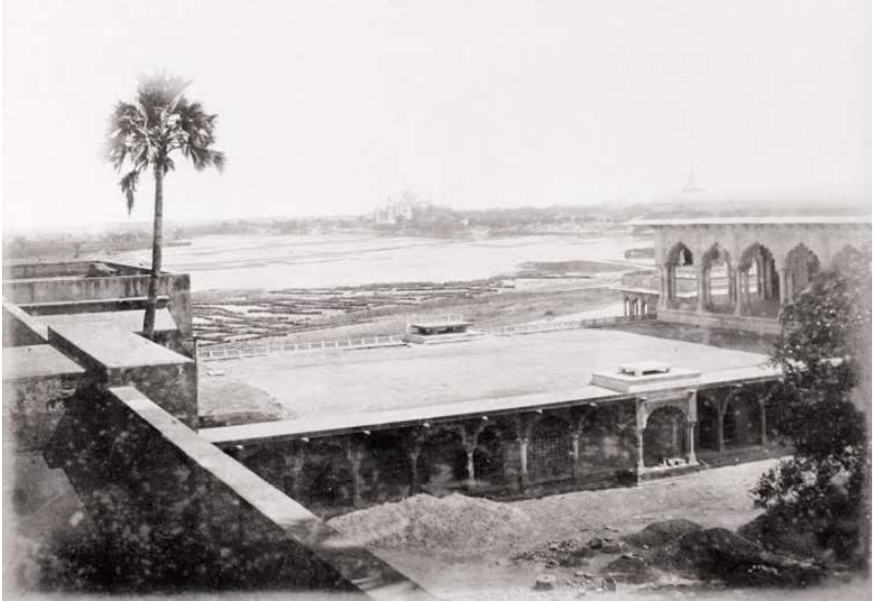
Image 15 A view of Diwan-i-khas taken from the north west, Agra fort, Source: Los Angeles County Museum of Art, Los Angeles, United States
