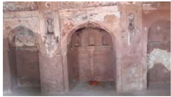
Figure 42: Plaster Delamination
