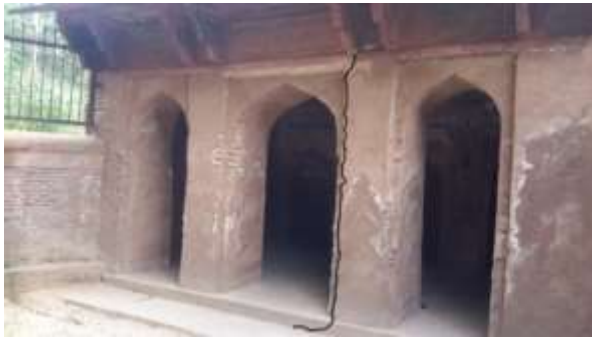
Figure 41: Vertical cracks
