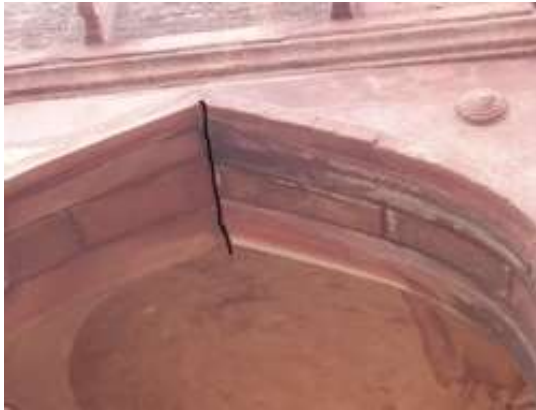
Figure 46: Structural Crack
