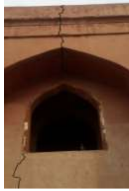
Figure 30: Vertical Crack
