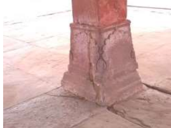
Figure 47: Wind Erosion
