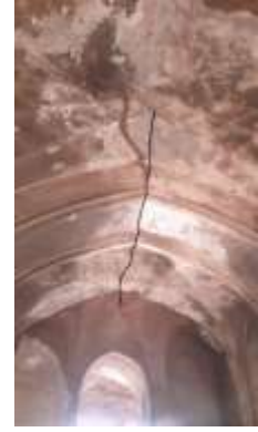
Figure 26: Horizontal Crack
