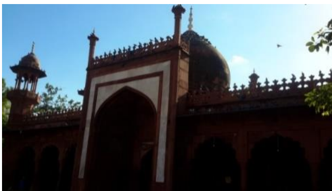
Figure 5.2.17 View of Fatehpuri Mosque
