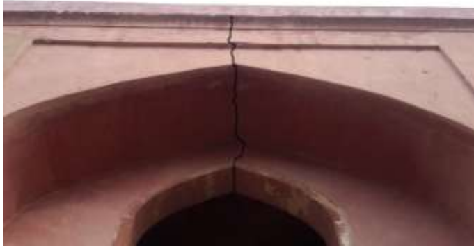
Figure 32: Structural crack
