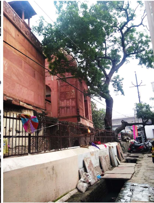
The rear view of the tomb with drainage nala along boundary wall
