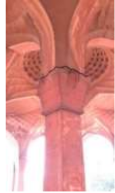
Figure 45: Horizontal Crack
