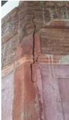
Figure 36: Vertical Crack
