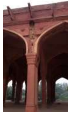
Figure 44: Vertical Crack
