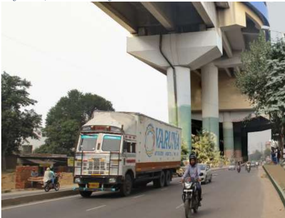
Image: SKV1 | View towards main gate of Akbar's Tomb from NH19 with visualisation of proposed Metro work
