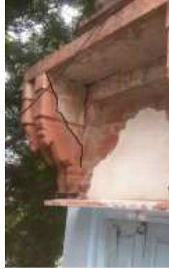
Figure 38: Structural Crack
