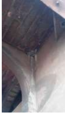
Figure 55: Moisture ingress
